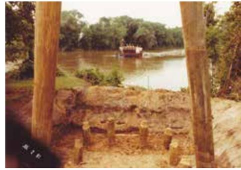
The Tridge was designed by Commonwealth Associates based out of Jackson, and built by Gerace Construction, which is based in Midland. The bridge consists of three wooden arches (weighing 44,000 pounds) that are supported by a single concrete pier, which also supports three 8-foot wide decks.
